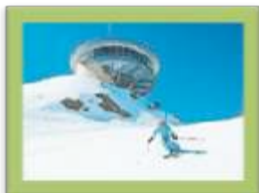
Upper Lift Restaurant
